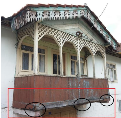
Figure 27: Oriel and wooden blocks.
