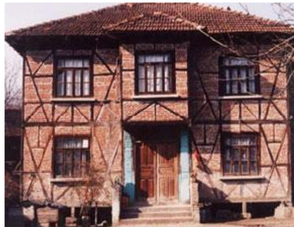
Figure 1: “Hımiş” wall structure.
