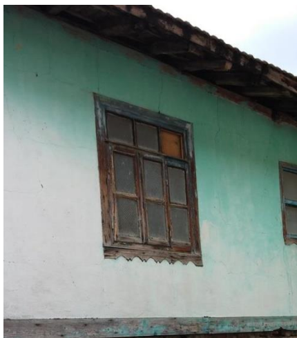
Figure 26: Windows and wood structure.
