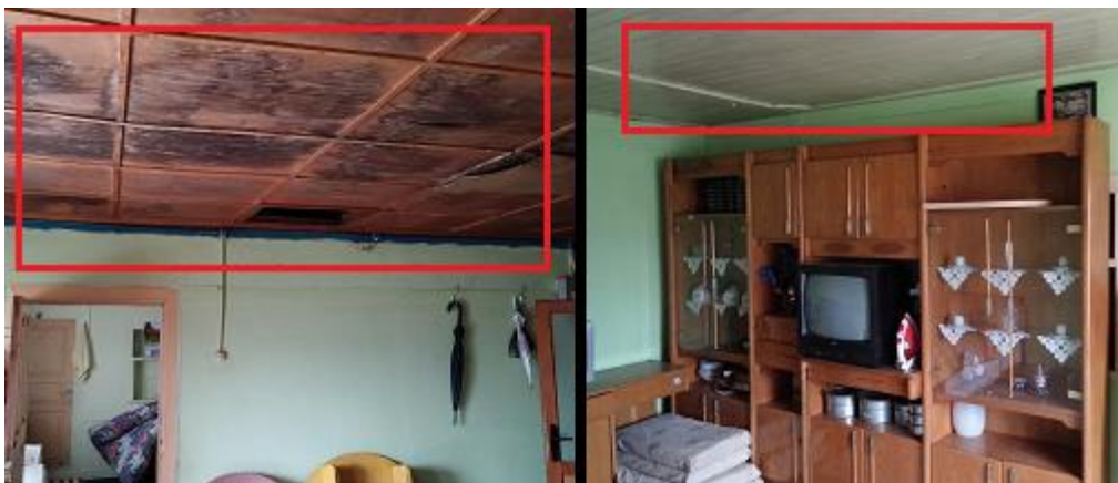
Figure 30: Wooden covered ceiling.
