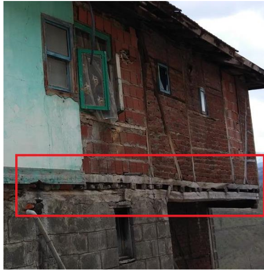
Figure 25: Space between wooden structures.
