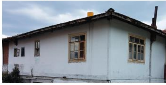
Figure 41: Shade effect of roof extension.
