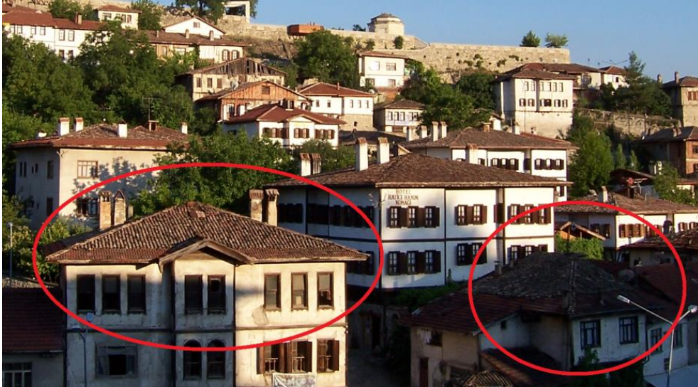
Figure 3: Examples of roofs from Safranbolu Houses.
